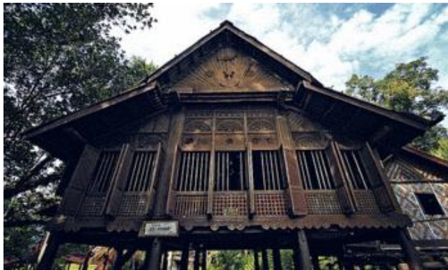
Fig. 6: The Non-Structural Components of Traditional Malay House similar to Vernacular Masjid building facade
