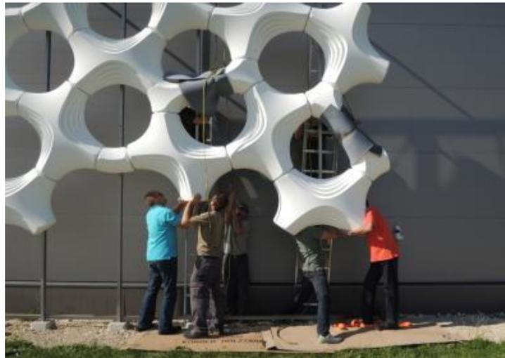
**Fig .3. Installation of the prosolve tiles [13]**
