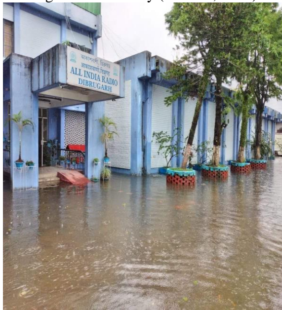
Fig9. Radio Centre (June 25, 2020)
