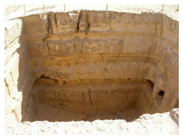
Figure 1. Photograph showing the erosion morphology on the southern wall of Campbell's tomb. Photograph courtesy of Jon Bodsworth (<u>http://www.egyptarchive.co.uk</u>).
