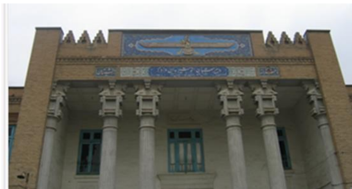
Figure 1 The Southern Façade of Anoushiravan High School (Source: Building Restoration Plan, 2013)
